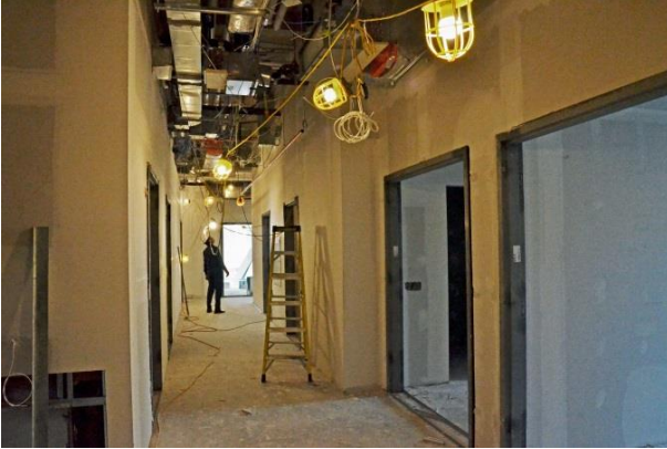
Yee Hong P K Kwok Hospice under construction
